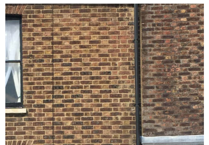
Photograph of 'speckled' brickwork in King's Lynn
