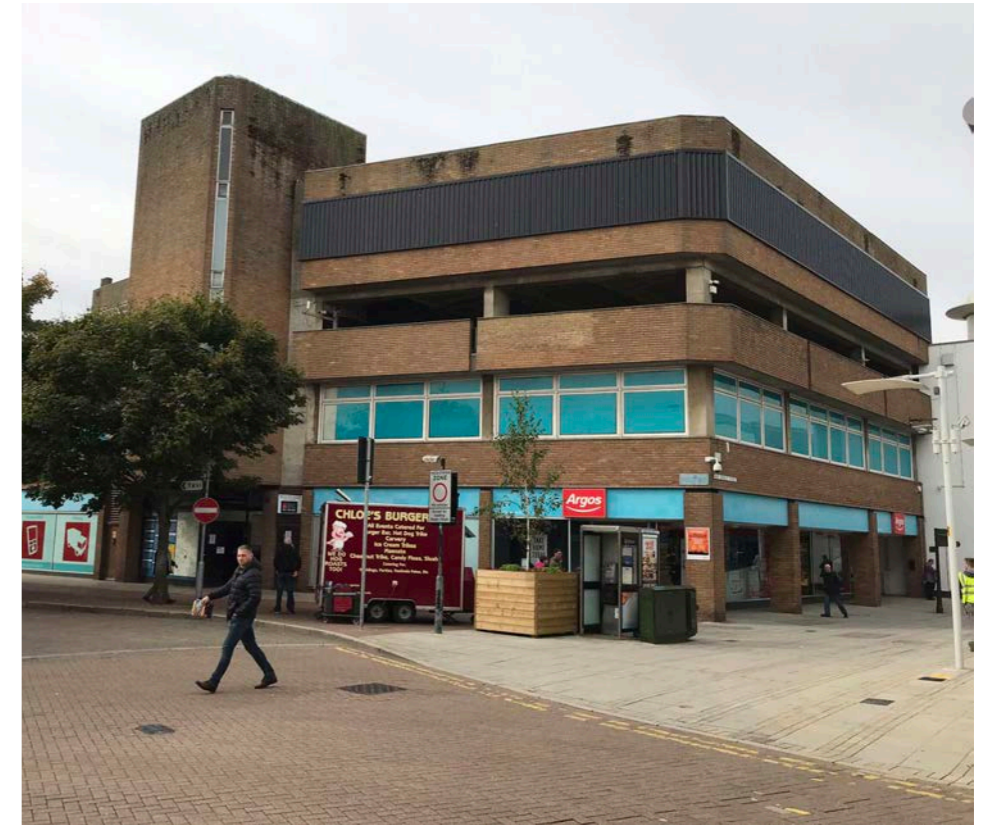
Photograph of the Argos building from Baxters Plain
